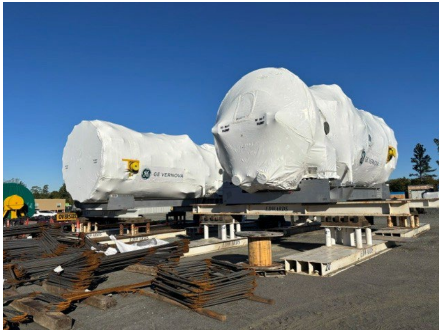
Photo 1: CC-1 gas turbines in site storage area
